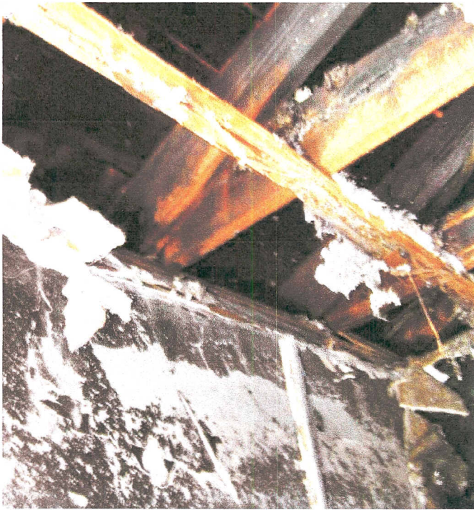
IMG_4288: Severe truss damage.
