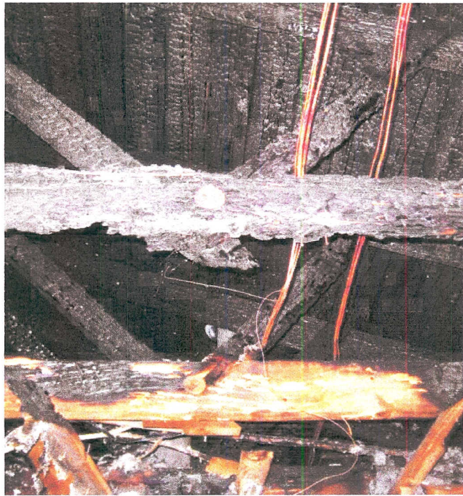
IMG_4289: Severe truss damage.
