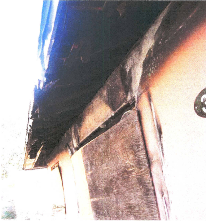
IMG_4304: Severely damaged trusses & roof deck.
