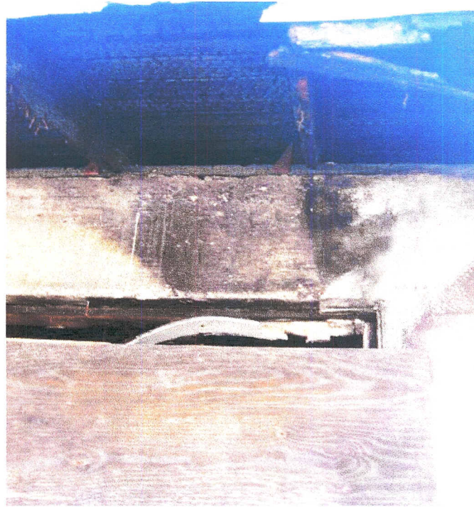
IMG_4305: Severely damaged trusses & roof deck.
